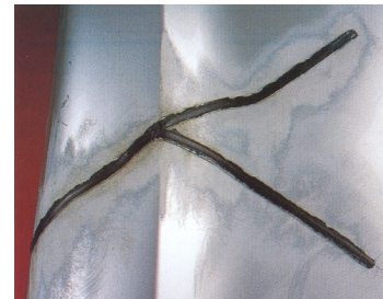
Completed Weld ready for finishing and painting
